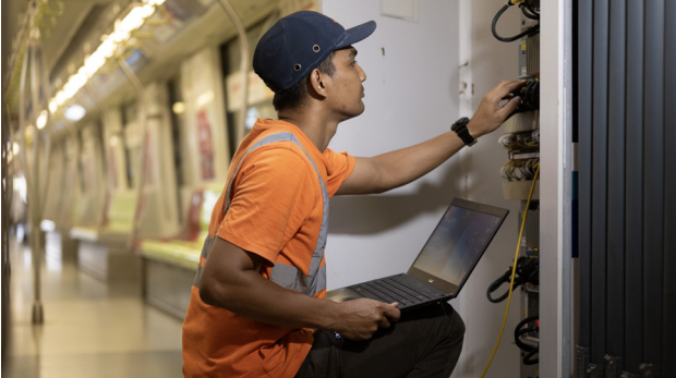
An SBS Transit rail technician conducting checks on a DTL train.
